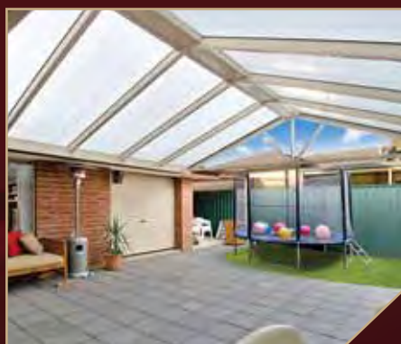
• Gable with Flat Polycarbonate sheeting
