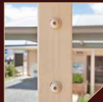
• Improved fixing method using painted stainless steel bolts
