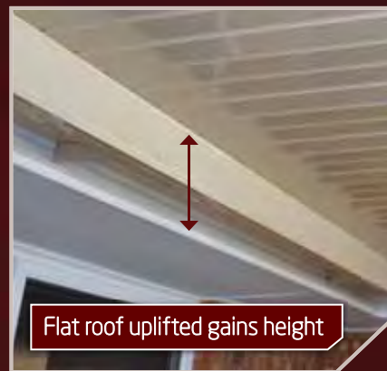
Flat roof attached to fascia
